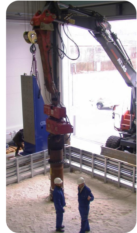
Vibration driven pile
