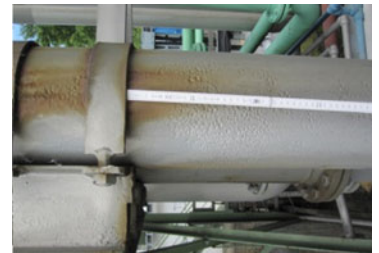
Fig. 2: Corrosion damages on pipes
