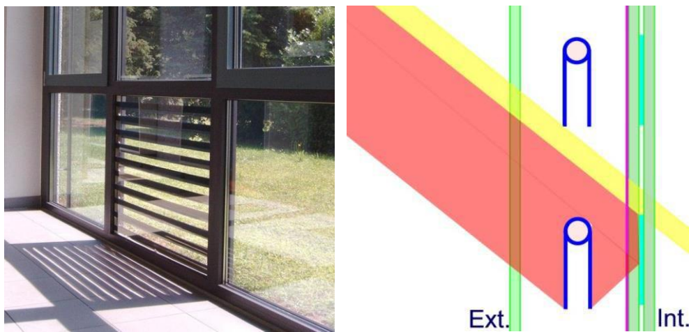
Figure 8: Collector from Robin Sun that uses reflection from the second glass pane [46]
