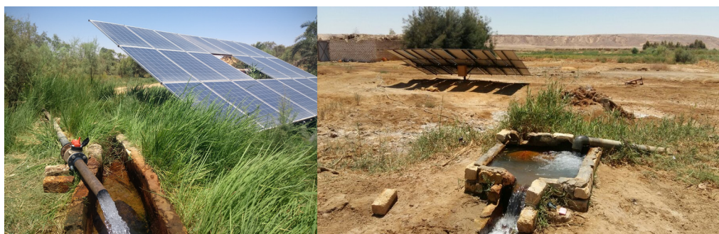
Fig. 6 Examples of solar PV pumps installed in the oasis of El Heiz, in Egypt’s Western Desert (source: authors).
