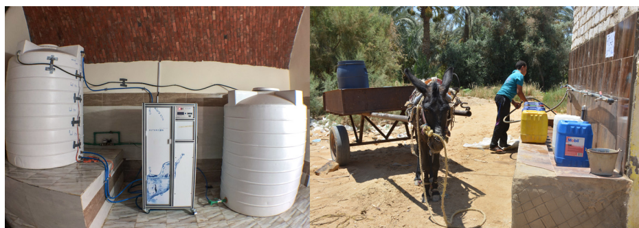
Fig. 8 Water purification system working on solar energy and using anodic oxidation for drinking water purification installed in Egypt's Western Desert (picture source: Kohler for AUC, 2018; authors, 2016).
