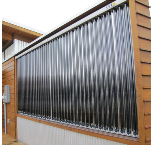
Figure 3: Proprietary evacuated tube array installed in BIST format
