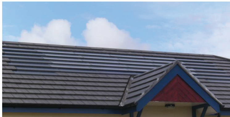
Figure 1: Combined BIPV and BIST roofing systems that offset traditional roofing material costs
