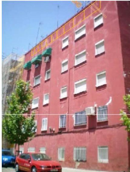
Figure 2: The demonstration building before refurbishment. The yellow frame at the top of the facade marks the area where the PVT component will be installed.
