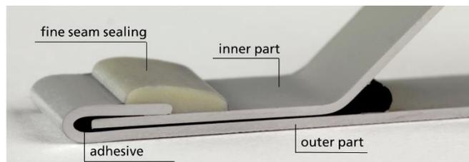
Fig. 2. Structure of a bonded hem.
