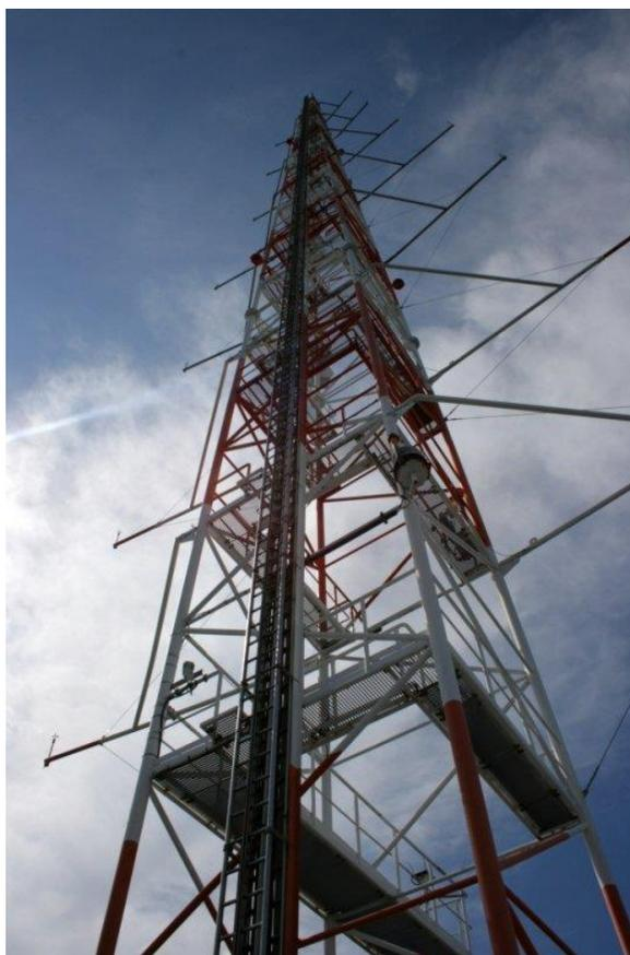
**Figure 1.2: Offshore met. mast FINO1 in the North Sea at the location N54 00' 53,5" E 6 35' 15,5". FINO1 measures among other things the wind speed, wind direction, air temperature, atmospheric pressure, atmospheric humidity and precipitation. The wind speed is retrieved at 100 m height and further lower heights [15].**
