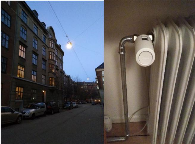
Figure 89. Picture of one of the test buildings and the thermostat prototype with the return temperature sensor.
