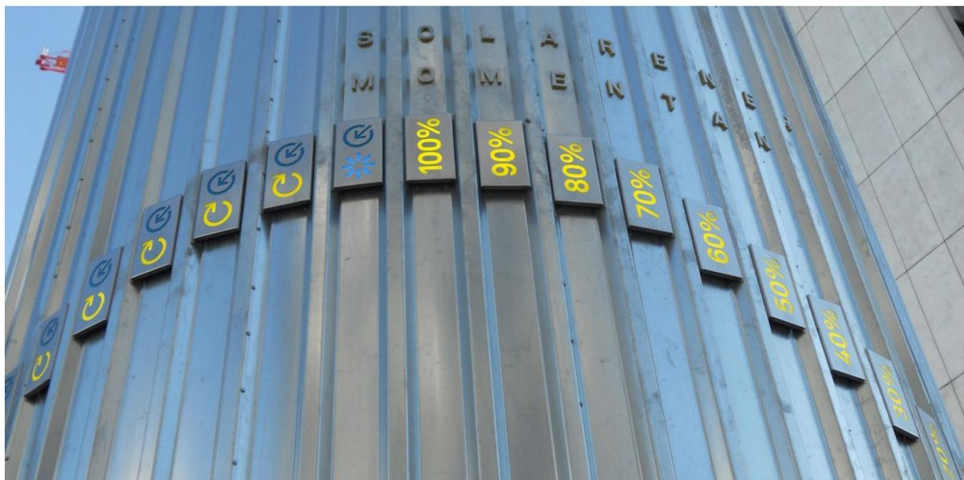
Figure 80. An LED visualisation on the buffer tank informs all passers-by how much thermal energy and how much electricity is currently produced by the sun and how much of the demand has been supplied in the last 24 hours (© SIR Strassl).
