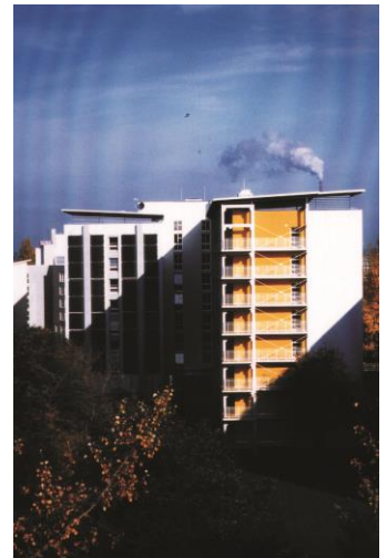
Fig. 4: One building wing shading the solar collectors on another façade of the same building, source: [12]
