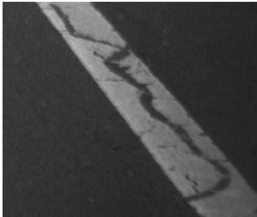
Figure 7. Example for poor marking quality, which results in lower SNR
