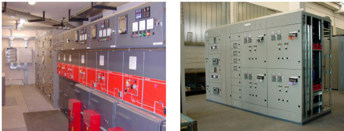
Figure 2: MV and LV supply, switching and interconnection boards at CESI's DG-lab [3]
